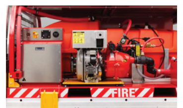
Electric starter kit for davey pump Pump isolation switch
