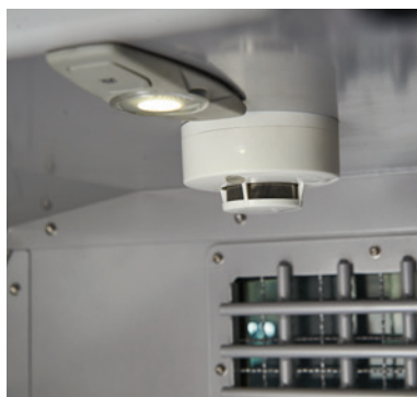
Dome light and smoke detector
